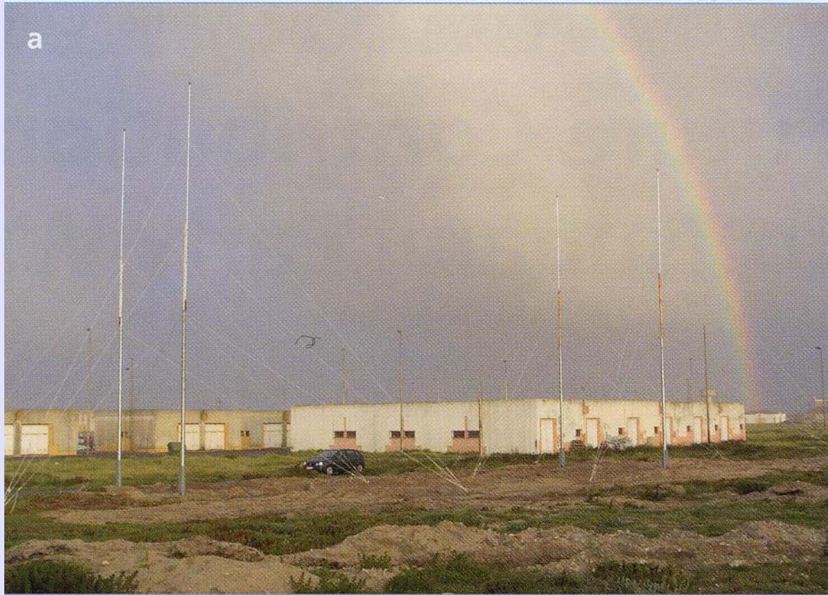
(a) the transmitting array
